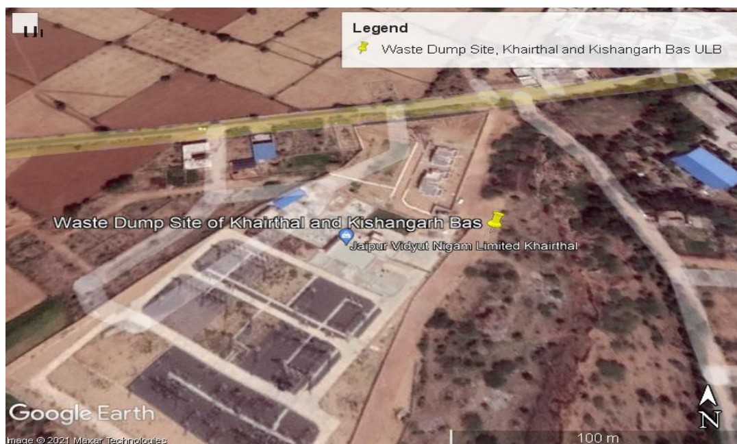
Figure 4.61 Waste Dump Site, Khairthal and Kishangarh Bas ULB (Coordinate 27°48'32.8"N 76°37'33.9"E)
