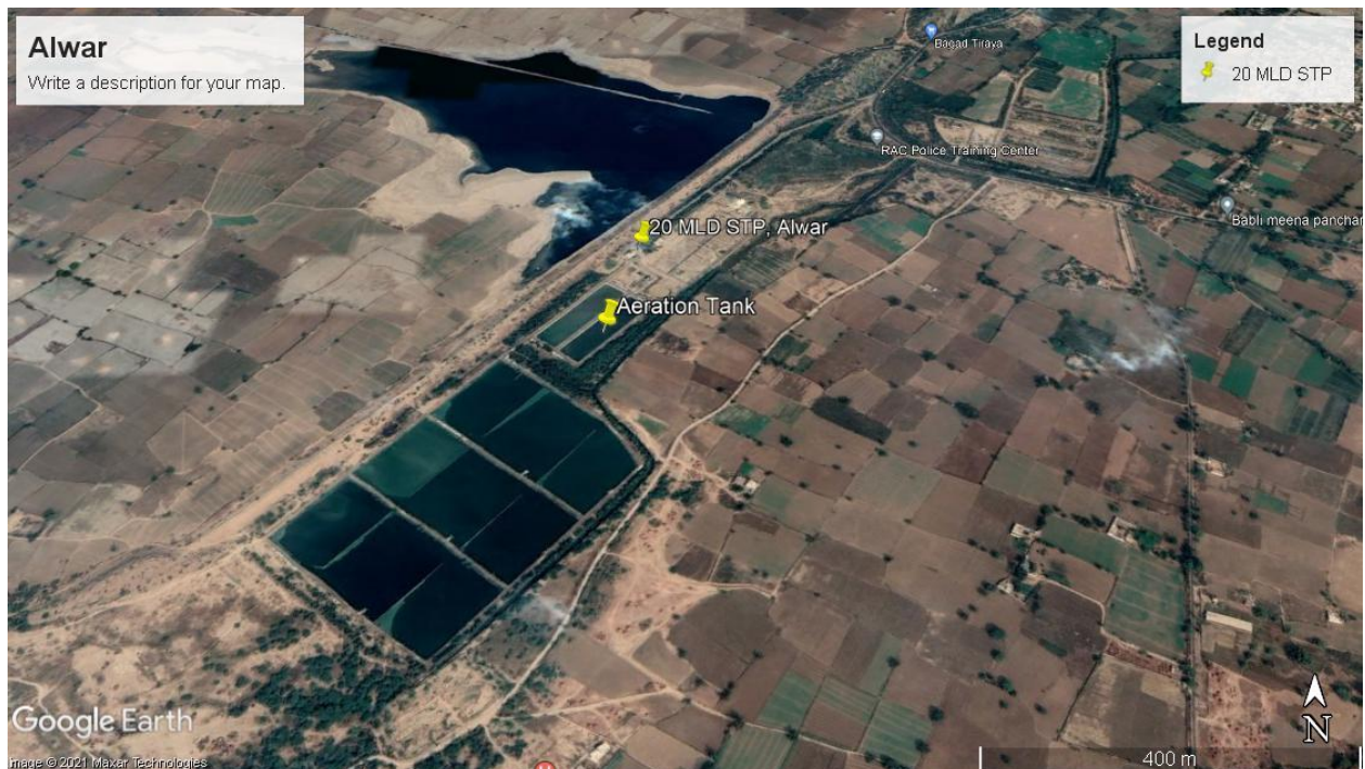
Figure 5.12 Google Earth view of 20 MLD STP, Alwar ULB
