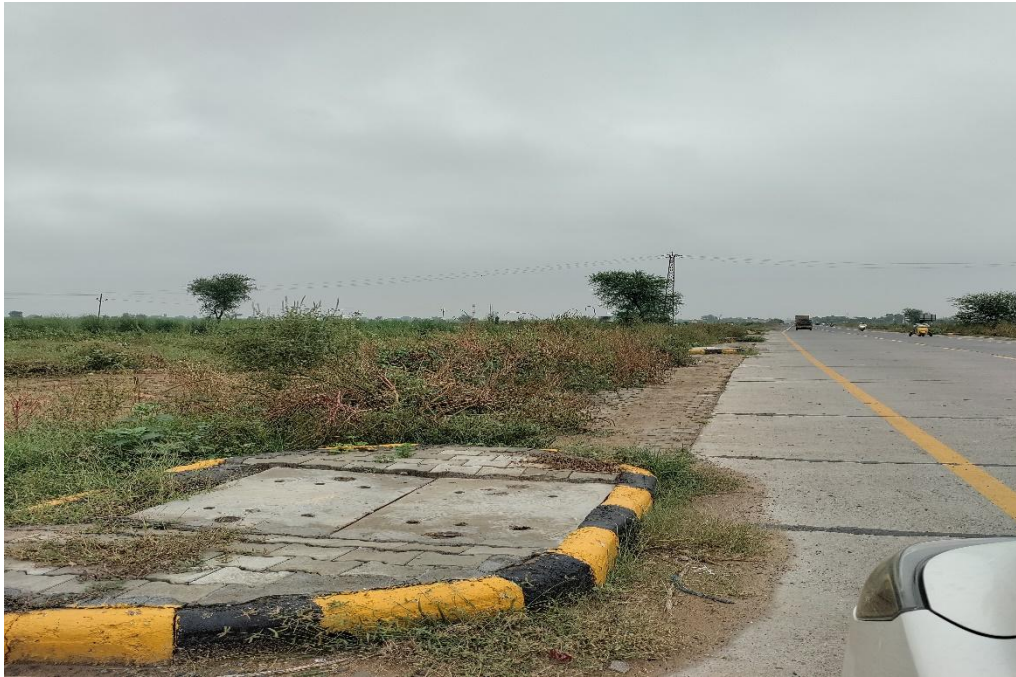
Figure 9.7 Road site Drainage work on Village Road (Coordinates- 27°34'01.5"N 76°47'36.2"E)
