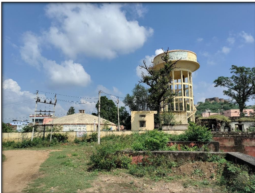
Figure 5.5 Overhead Water Supply Tank in Rajgarh ULB (27°14'08.8"N 76°36'41.8"E)
