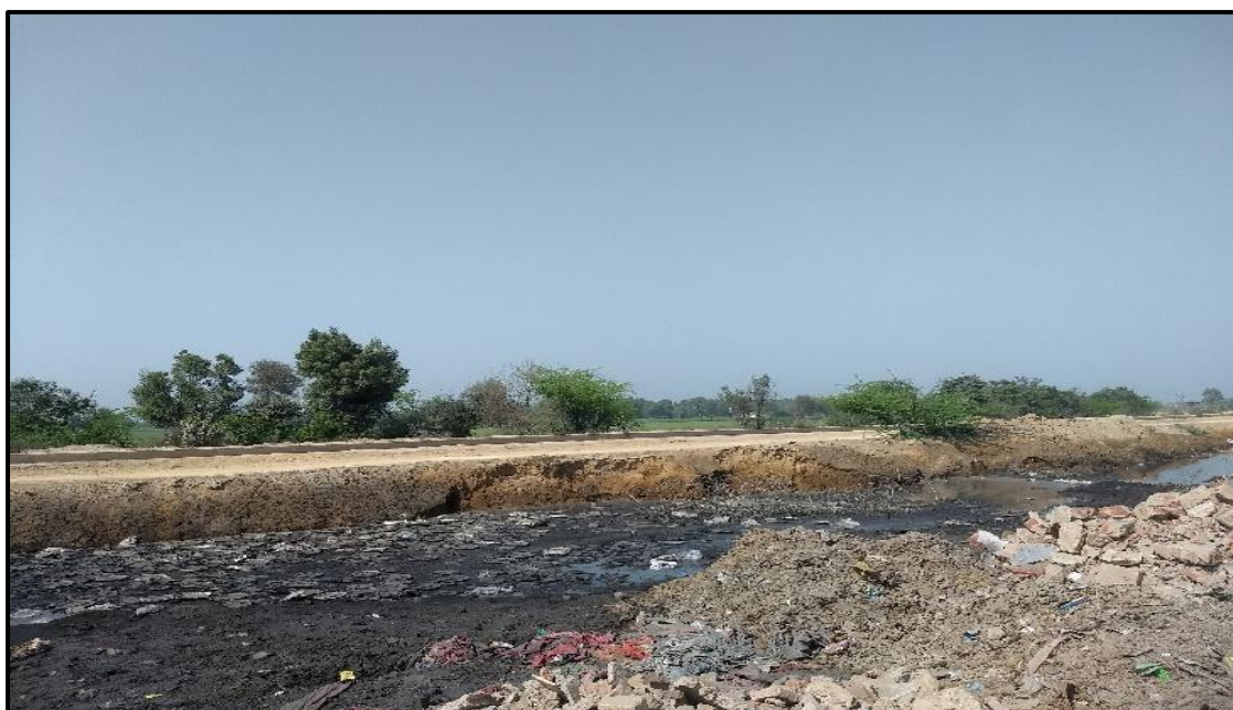
Figure 7.4 Stagnant untreated industrial waste water and accumulation of sludge
