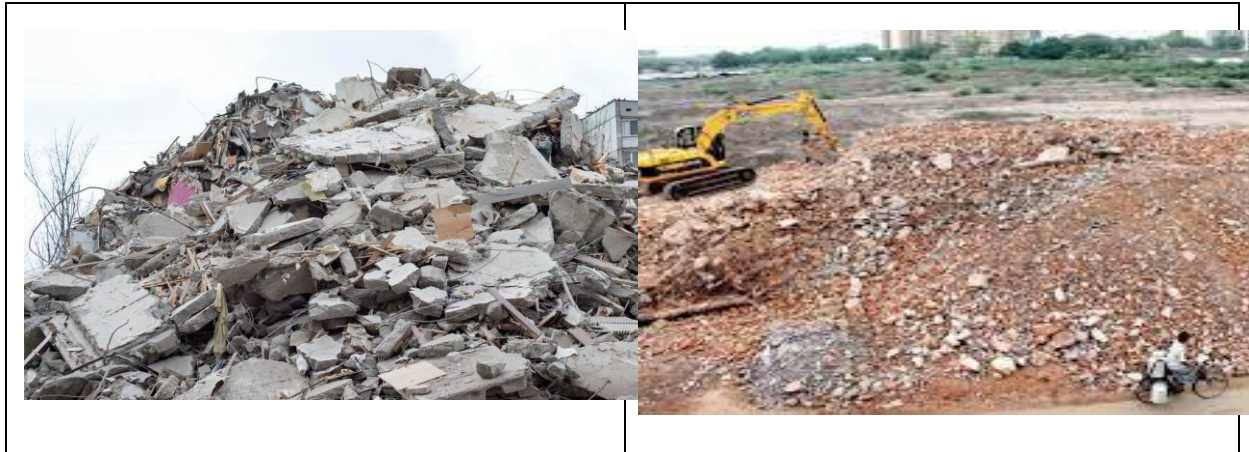
Figure 4.10 Construction and Demolition Waste
